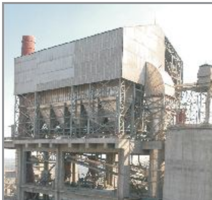
Cement Mill Bag Filter in a Cement Plant
