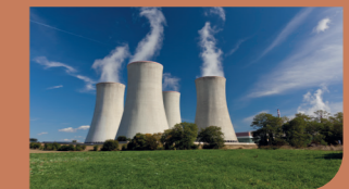
Power & Ash Handling
